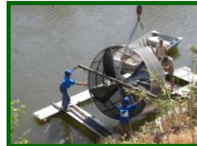
SPC and CDFG installing the TID screw traps at Grayson.
