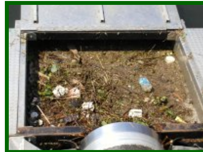
Debris accumulated in the livebox overnight during the high flow period.
